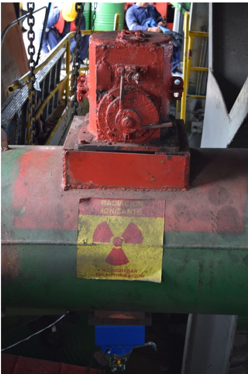
FIGURE 1. Radiation Source and Density Sensor (left), Flowmeter (right),
